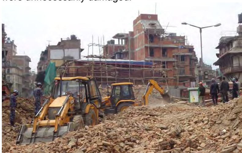
Fig. 1: Clearing debris at the Kasthamandap temple, Hanuman Dhoka Durbar Square.
