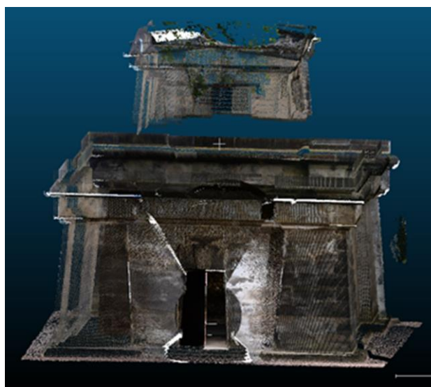
Figure 1. Part of the ground-based LiDAR survey of Trentham Mausoleum, Stoke-on-Trent, UK.
