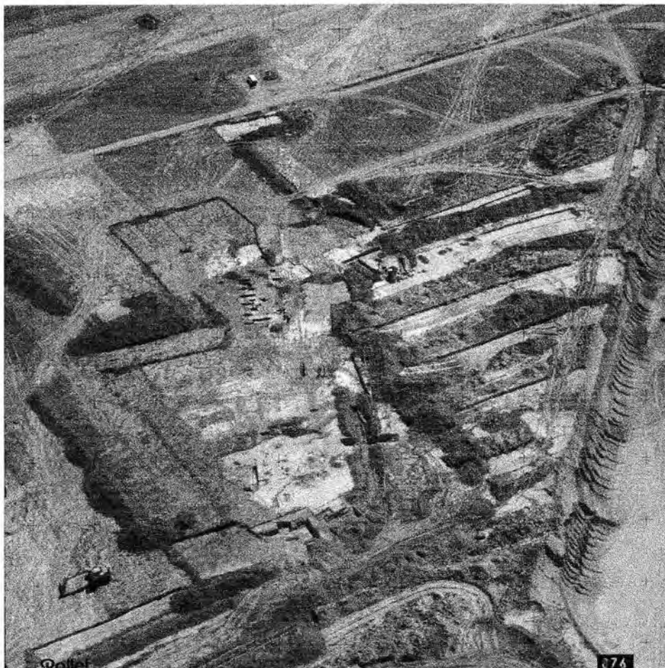
Fig. 3. Excavation on the site short before cole-mining comes (A03286/MSBE95 LVR/RAB/Zantopp, R.)
